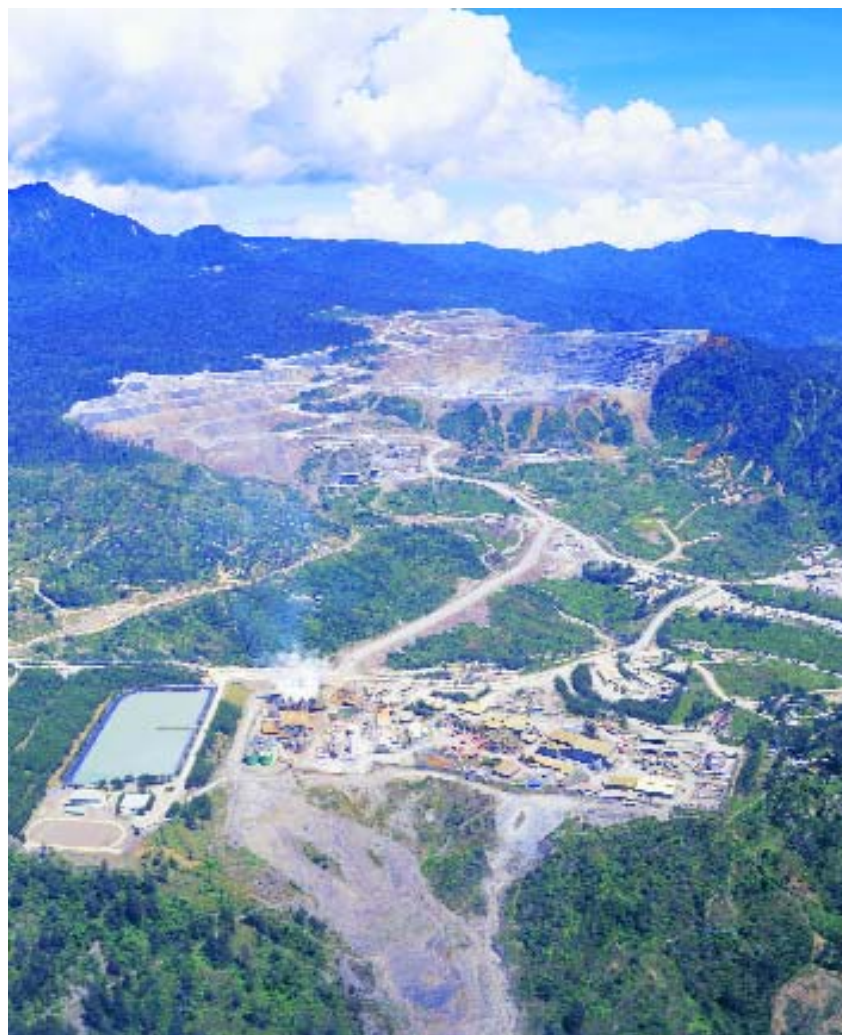
Porgera mine and mill
