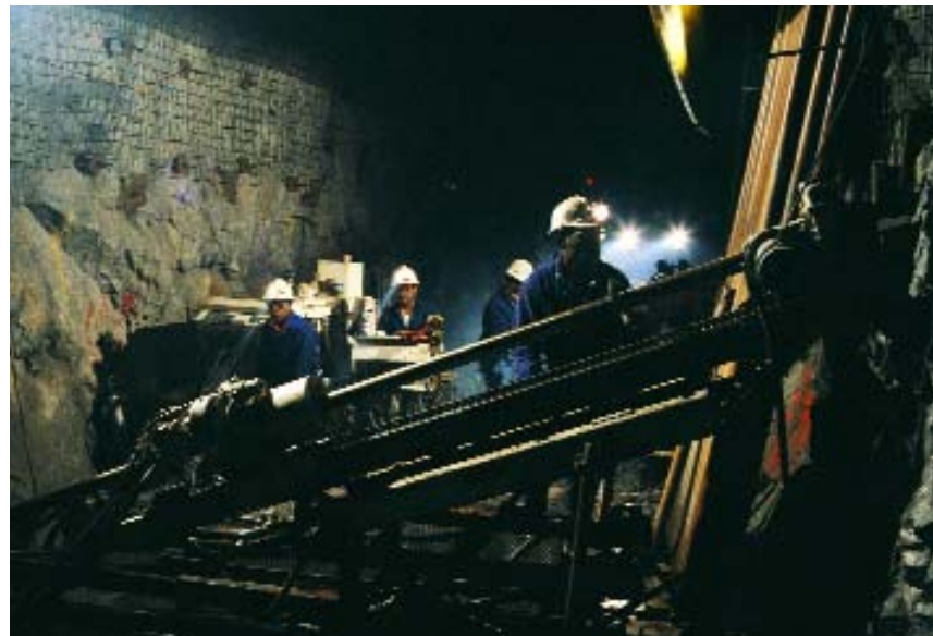
Underground stope preparation
